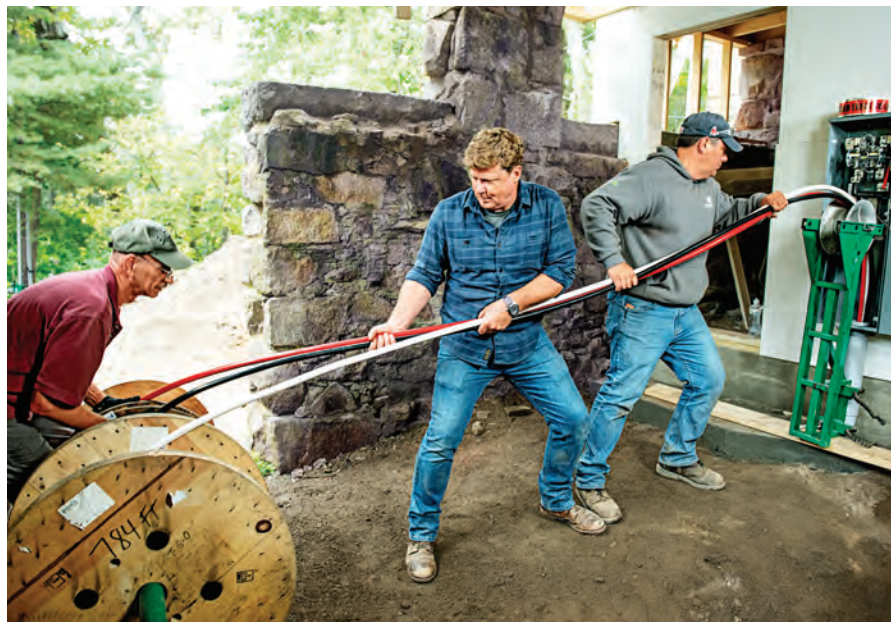
ABOVE: TOH host Kevin O’Connor, master electrician Heath Eastman (on the right), and George Lane of Eaton & Eastman Electric pull cable from spools for the house’s electrical service. The cables will be buried in a trench from the house to the street hookup.
